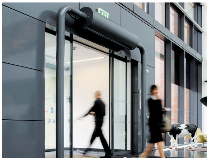
Rund Installation with special goalposts supports
